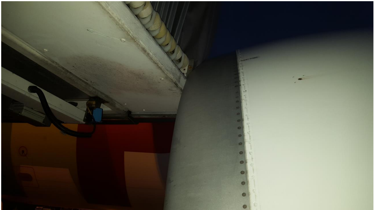
Figura 3 - Patamar exterior da ponte onde está instalado o mecanismo de auto-nivelamento || Figure 3 - The outer level of the bridge which is installed the mechanism of self-leveling
