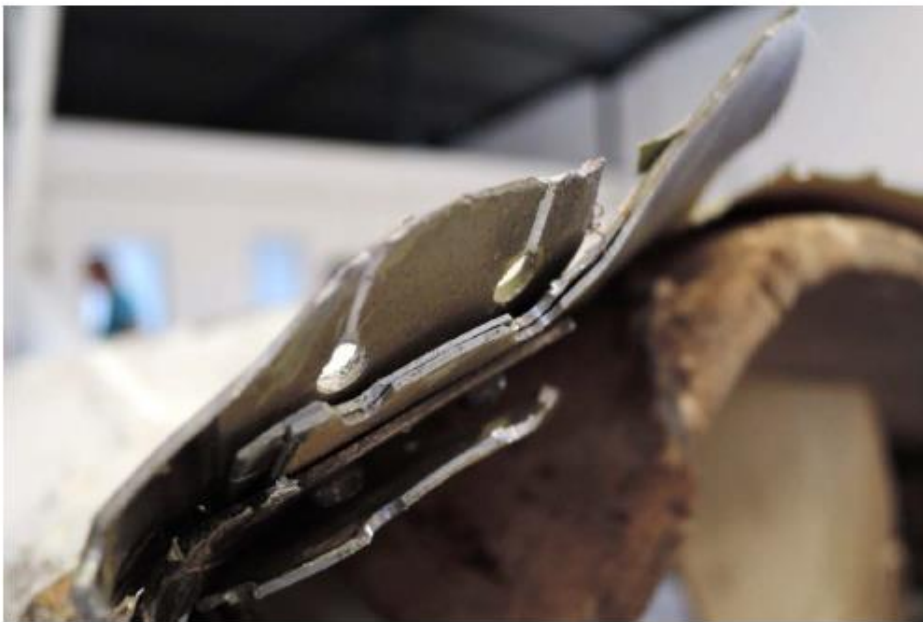
Figure 4: Appearance of a section of sample no. 2 during the visit in Viseu
