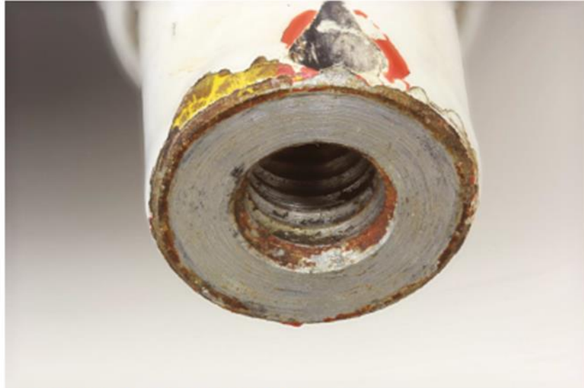
Figure 16: Condition of the thread at the RH rod (reference)
