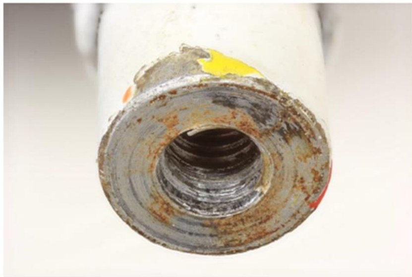
Figure 17: Condition of the thread at the LH rod
